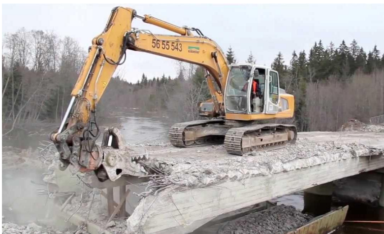
Figure 6: Bulldozer breaking a bridge
