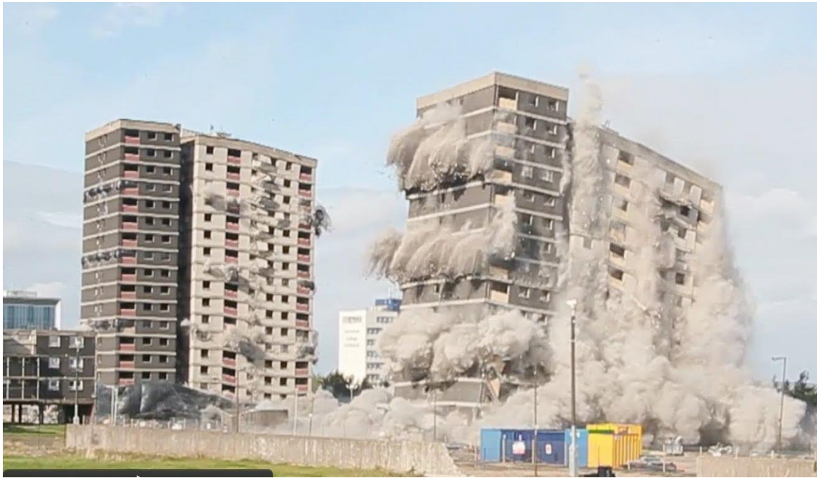
Figure 15: Implosive controlled demolition
