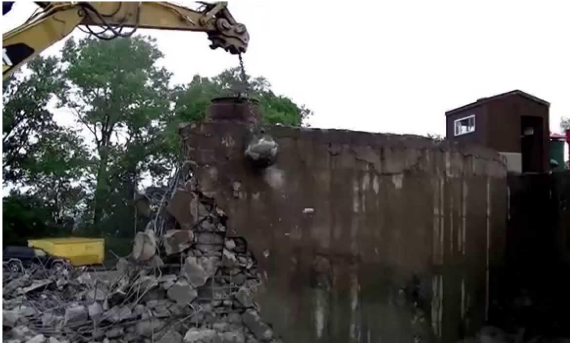
Figure 7: Wreking ball demolition
