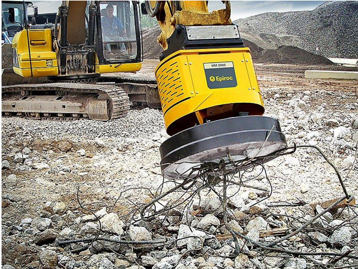
Figure 14: excavator with electro-lifting magnet
