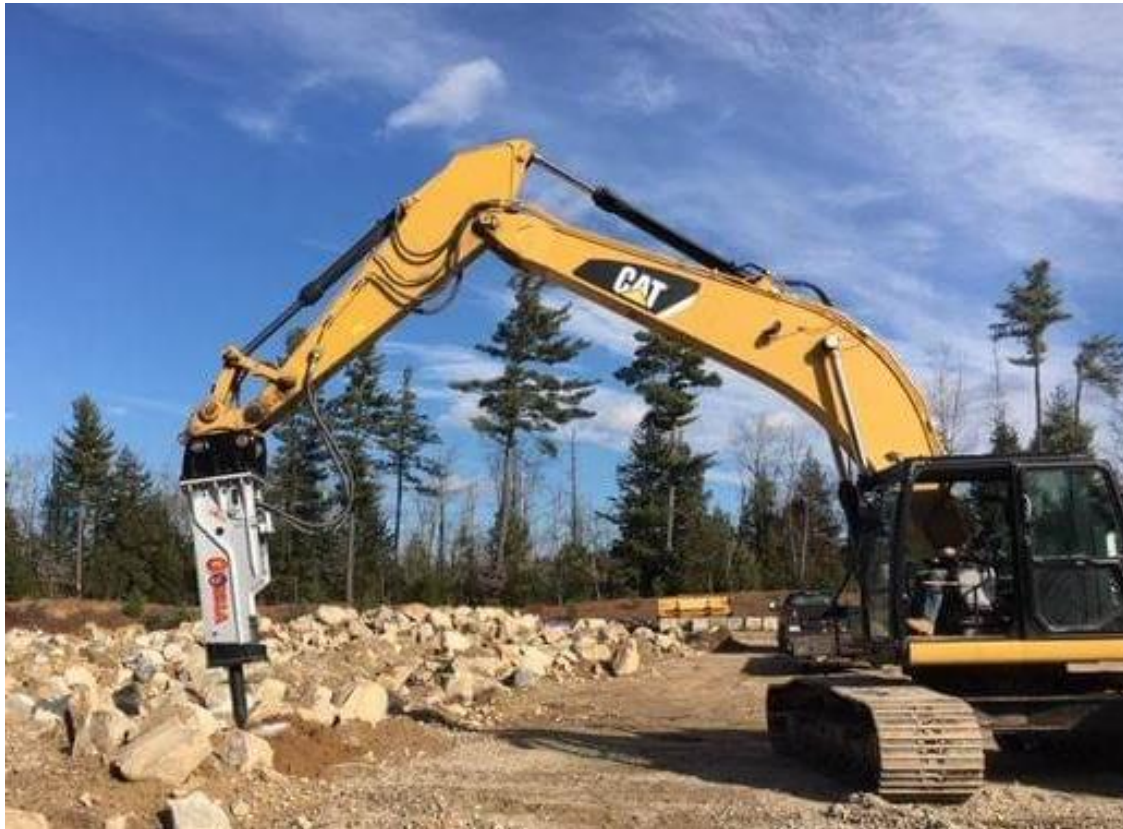
Figure 13: Excavator with hydraulic breaker
