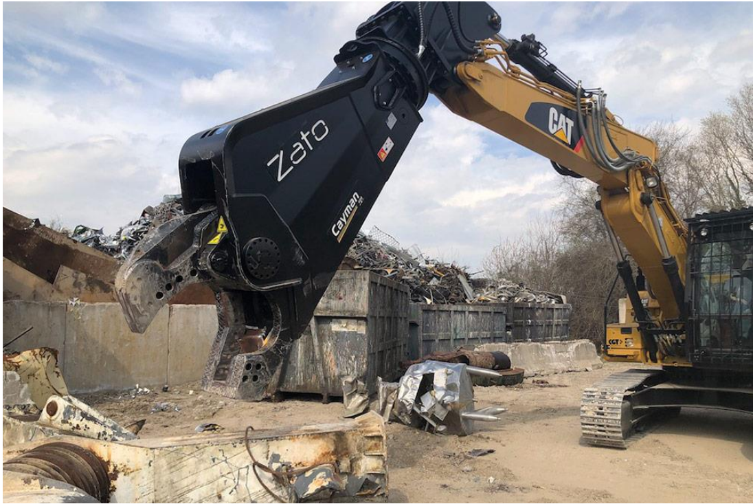
Figure 9: Excavator with demolition shear
