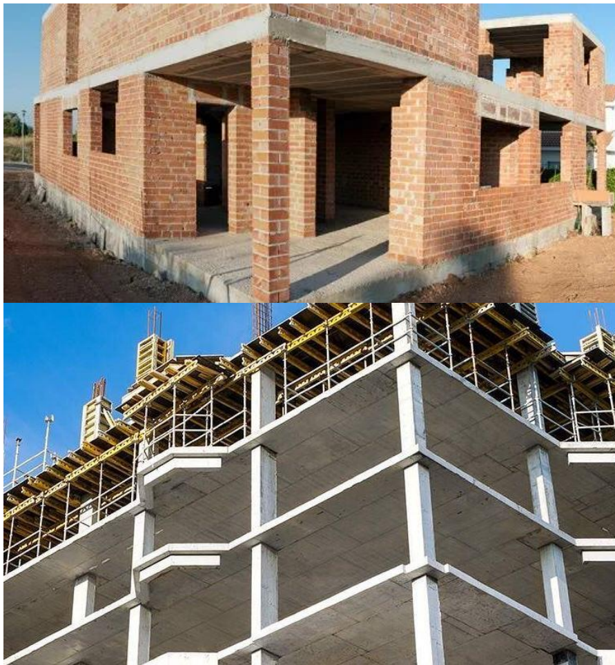
Figure 2: Buildings with concrete/masonry structure.
